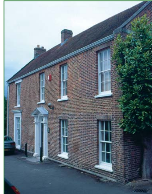
Secretariat offices at Dennett House, Taunton
